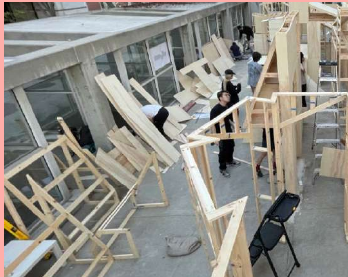
Image: Students installing the FRS, photography by students.
