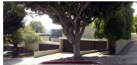
3, 4. Toward a new process: Avenel Cooperative Housing Project by Gregory Ain, Los Angeles, 1947. Top: Drawing by Stephen Crews and Samantha Gilk. Bottom: Photograph by Kansas Sebastian via Flickr, CC BY-NC-ND 2.0: https://www.flickr.com/photos/kansas_sebastian/4651758738/ .
