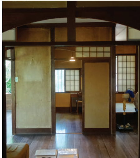
figure 28.12 Looking out from guest room into the living room, with engawa (left), study (front) and Tatami room (right) with operable transoms above each opening
