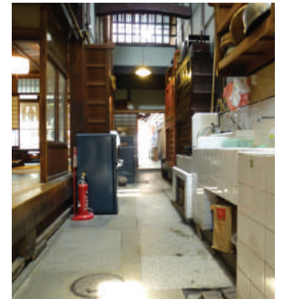
figure 28.8 Tori-niwa in machiya in Kyoto, raised floor and below floor ventilation space (lower left of the picture)
