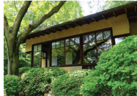
figure 28.9 Chochikukyo south façade, looking at the engawa
