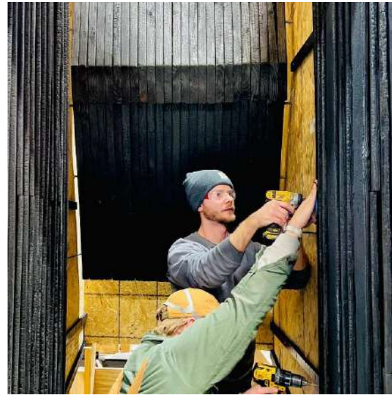
Images of UDBS students constructing a full-scale section mockup of Sensing the Forest, used to study details and understand logistics of constructing and cladding the structure.
