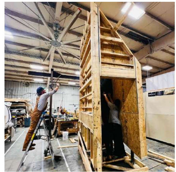
Images of UDBS students constructing a full-scale section mockup of Sensing the Forest, used to study details and understand logistics of constructing and cladding the structure.
