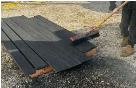
Students used a propane-fueled kiln and propane torch to apply the Shou-Sugi Ban finish on all exposed wood members.
