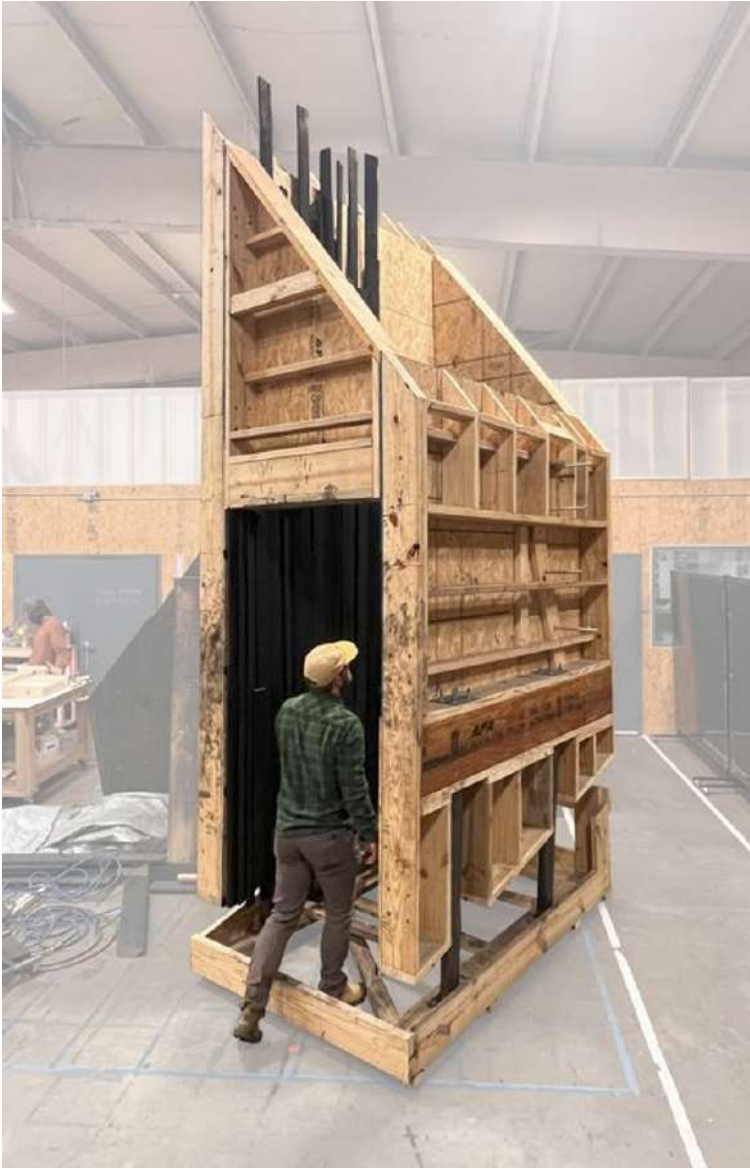
Images of UDBS students constructing a full-scale section mockup of Sensing the Forest, used to study details and understand logistics of constructing and cladding the structure.
