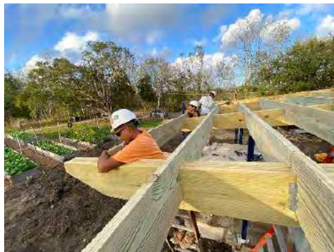
10. reinforce rafters with hurricane ties
