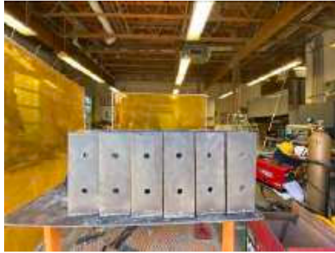
2. prefabricate column saddles
