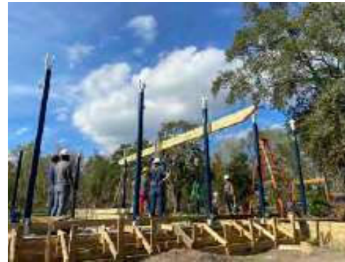
7. raise and install beams
