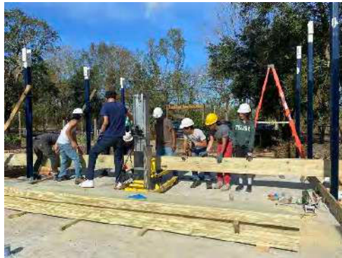
6. fabricate layered beams
