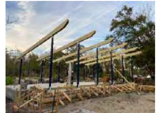
8. secure beams with structural bolts
