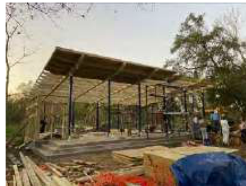
11. install plywood sheathing
