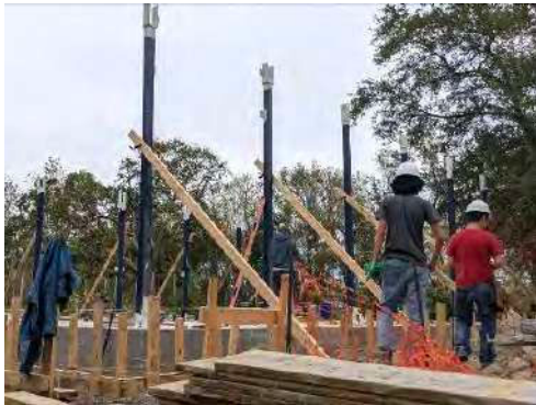
5. erect and secure columns
