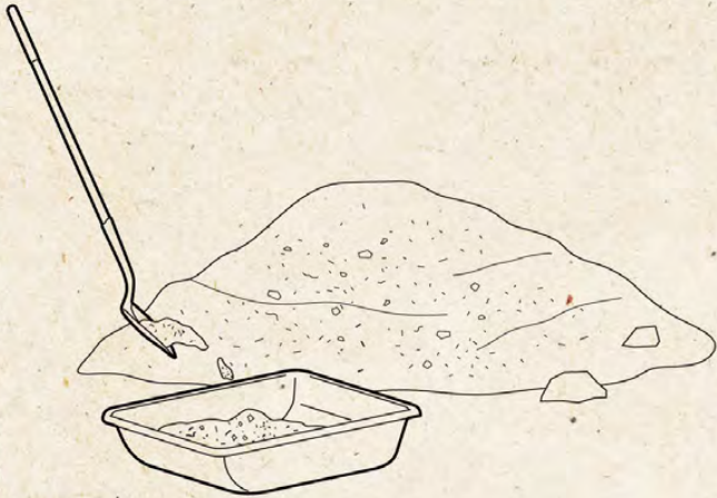
1 "Filling Station" Fill up the mixing tub with 2 shovels of sand, 8 shovels of clay, and 1 shovel of cement
