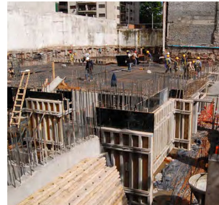
Construction visit - Buenos Aires
