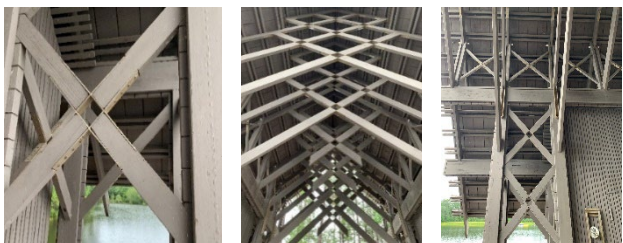
Pine Eagle Chapel at Camp Tiak - Wiggins, Mississippi by Fay Jones
