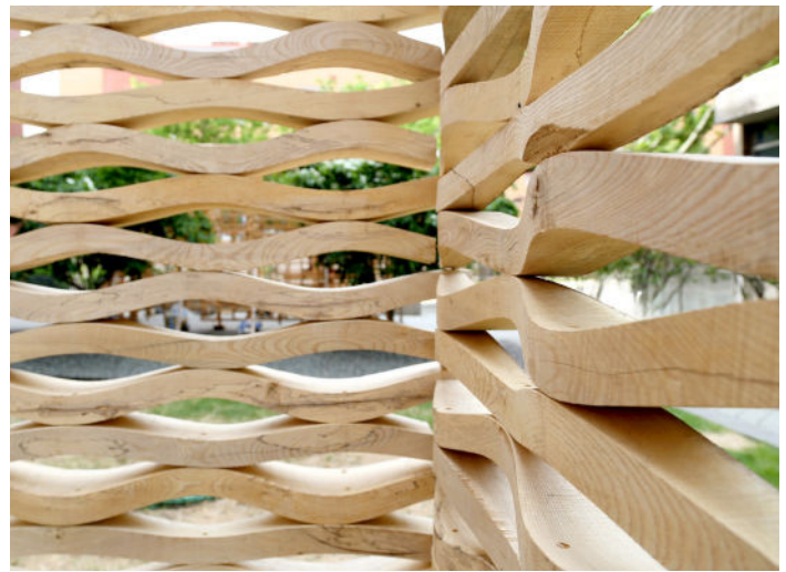
Detail of timber elements milled with the robotic sawmill technology and deployed in "Crinkle Cuts," a pavilion constructed by a workshop at NJIT.
