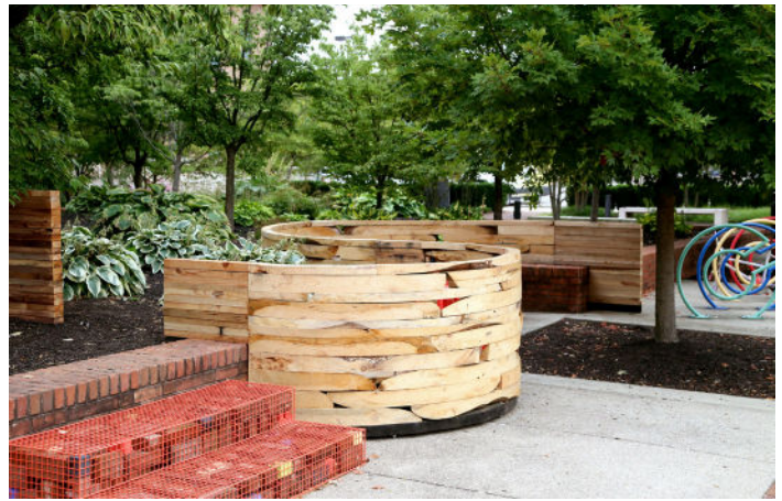
"Sylvan Scrapple" is a temporary installation built by a team of paid student researchers and displayed at Exhibit Columbus in fall 2023. It is the first work fabricated using the new robotic sawmill and represents one of the simplest possible applications of the sawmill technology.
