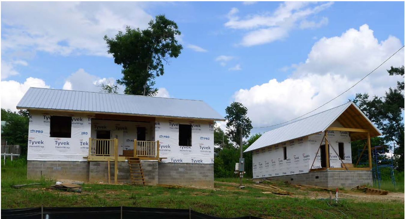
Figure 5. Pilot project under construction. Image credit Auburn University Rural Studio.
