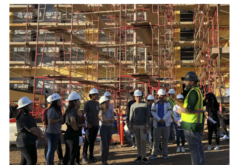
UHM Life Sciences construction site walk-thru
