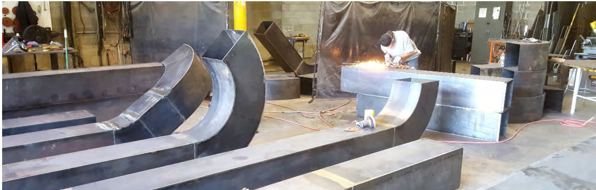
Fabrication in Shop
